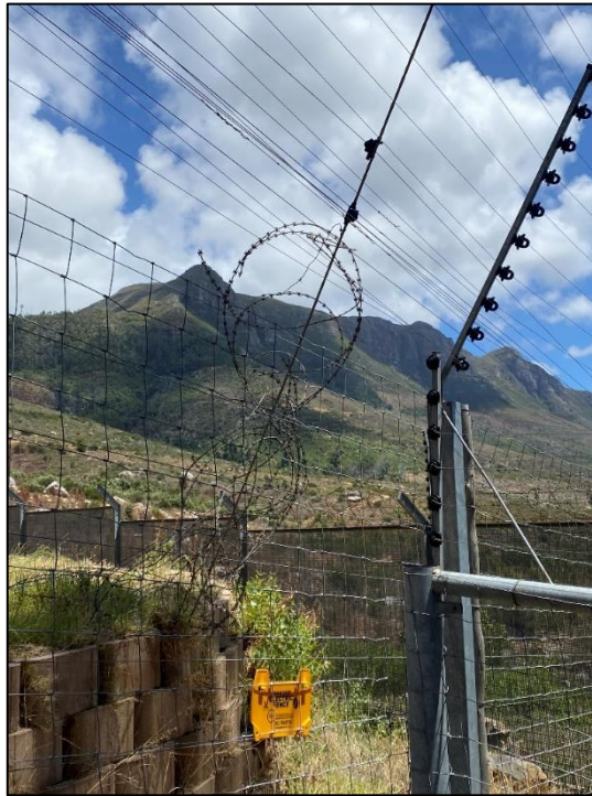
Figure 9. Razor wire used to prevent baboons from accessing Zwaanswyk via tower anchor wires.
